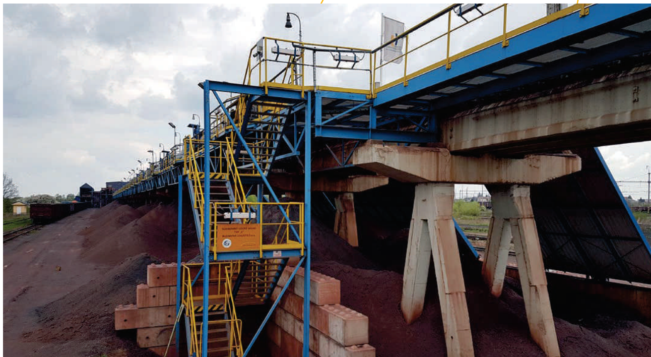
Skladová plocha pod III. Vysokou rampou – colný sklad. Storage area below the 3rd High Ramp - customs warehouse.
